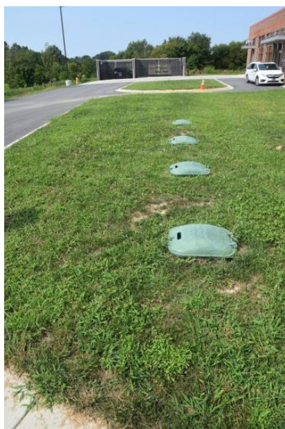
Underground Propane Tanks
