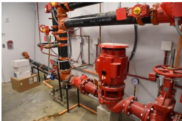
Main Fire Service main with Fire Pump
