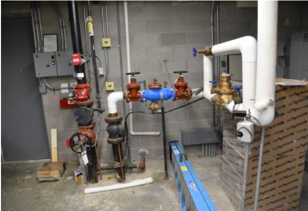
Water Service and Fire Service
