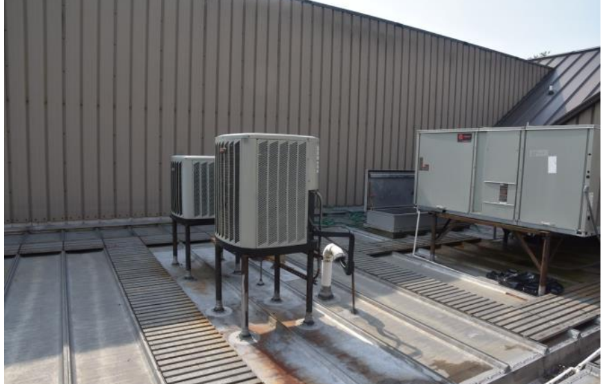
Condensing unit near wall for meeting room fan coil
