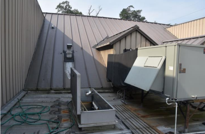
Rooftop unit "E" and exhaust gooseneck
