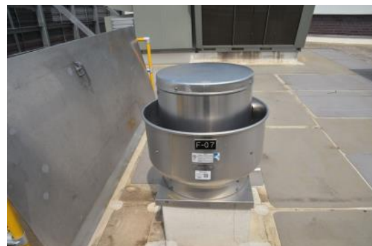
Typical Exhaust Fan on Roof
