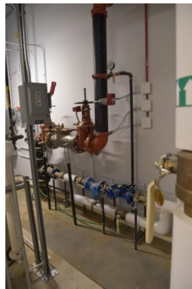
Water Service and Fire Service
