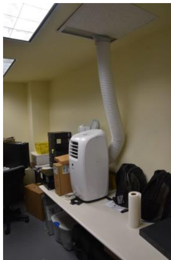
Portable Cooling Unit
