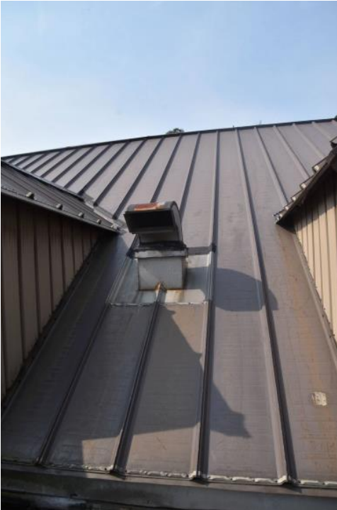
Outside air intake for fan coil units.
